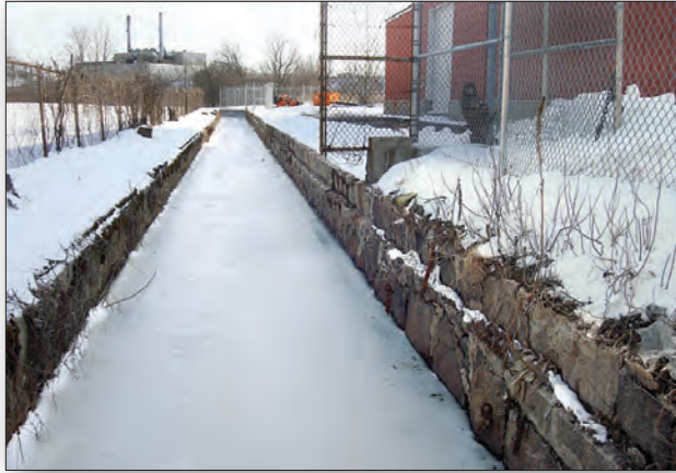
A man-made sluiceway directed water from the Quequechan River into the mills to be used for steam power.
