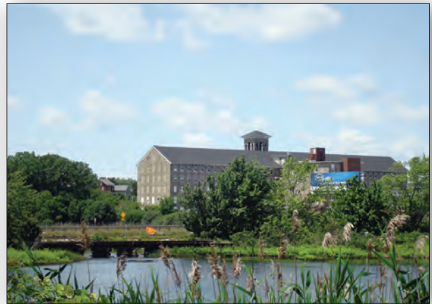
An old railroad bridge crosses the Quequechan River near the Crescent Mill (built in 1872), 2009.
